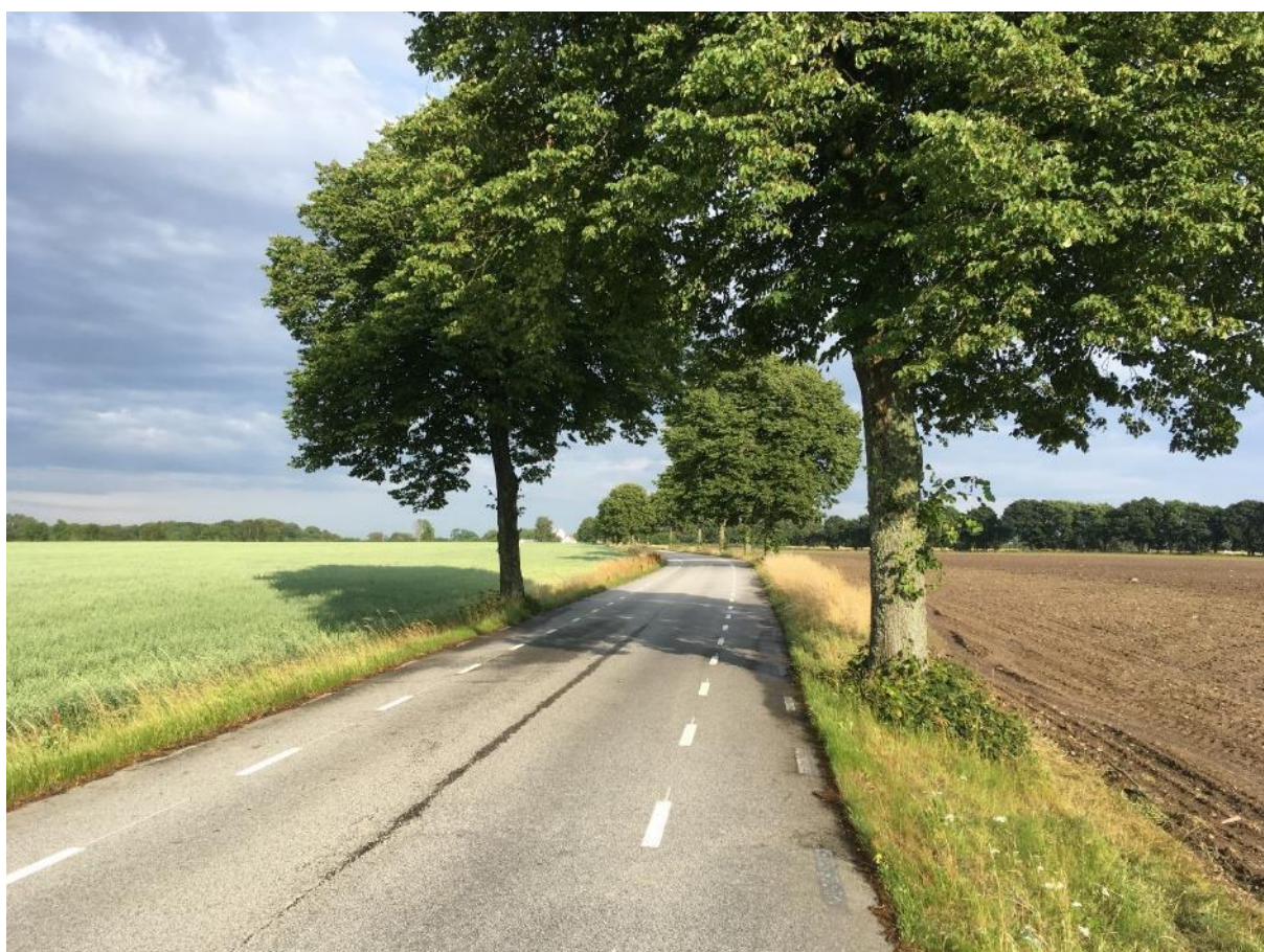
Figure 13: 2-1 road in Sweden with a central, share lane for both traffic directions. (Source: © UFO-monumentet, https://commons.wikimedia.org/wiki/File:Bygdev%C3%A4g.jpg license: https://creativecommons.org/licenses/by-sa/4.0/deed.en ; No modifications)
