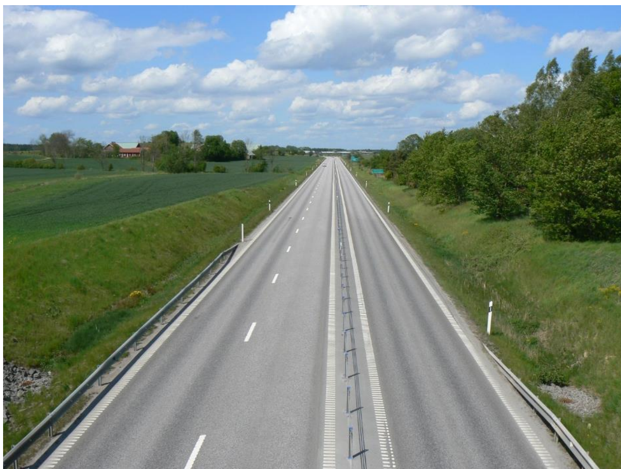
Figure 11: 2+1 road in Sweden with a physical separation between the opposing driving directions. (Source: https://commons.wikimedia.org/wiki/File:MMLNorr1.JPG )
