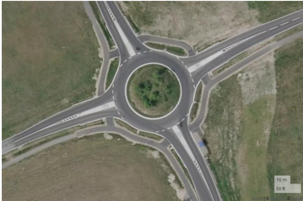
Figure 16: Non-urban roundabout. (Source: created using https://geojson.io © Mapbox (see: https://www.mapbox.com/about/maps/ ) © Maxar (see: https://www.maxar.com/ ))
