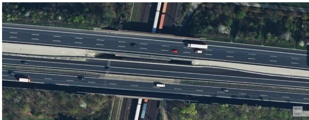
Figure 5: A split of the motorway A2 as aerial image, close to Lehrte. (Source: created using https://geojson.io © Mapbox (see: https://www.mapbox.com/about/maps/ ) © Maxar (see: https://www.maxar.com/ ))
