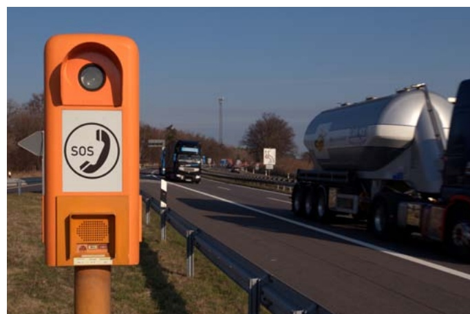
Emergency telephones with their distinctive appearance are mounted in a constant distance of about 2000 meters on both sides of German motorways, on its ramps and exits. The ANIKA projects aim at extending them to cooperative ITS road side stations.
